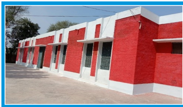
Rehabilitated classrooms of Gul wala, Alipur, Muzaffargarh
