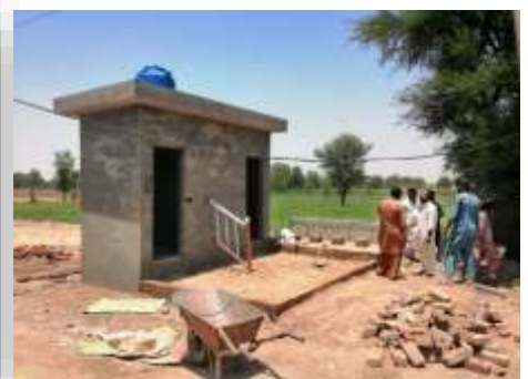
Figure 8: LPP technical team while overseeing public toilet construction site
