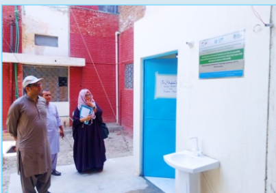
Construction of toilet in Govt technical training institute Bahawalpur
