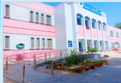
Ramps construction in Govt Technical institute Bahawalnagar
