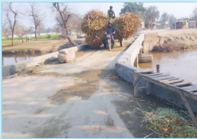
Bridge construction Munshi wala Lodhran 2024
