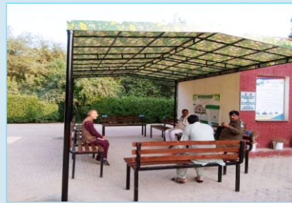
Installation of shed in Police station Kehrur Pacca Lodhran
